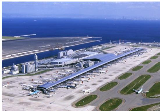
The terminal's roof is shaped like an airfoil. This shape is used to promote air circulation through the building: giant air conditioning ducts blow air upwards at one side of the terminal, circulate the air across the curvature of the ceiling, and collect the air through intakes at the other side.
